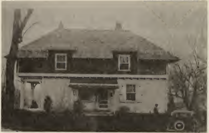
Figure 61. Caretaker's house designed by Herbert Johnson Wetherill. (Wetherill-Parker Family Private Collection)
